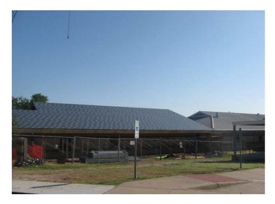
This is a view of the AMCMS after roof insulation and waterproofing underlayment have been installed.
