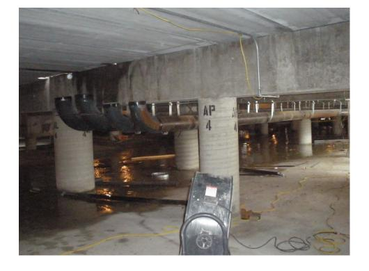
This is a view from below the deck planks in the crawl space. You can see the chilled water piping that is hanging from the concrete beams, which will carry chilled water to the multiple air handling units throughout the building.
